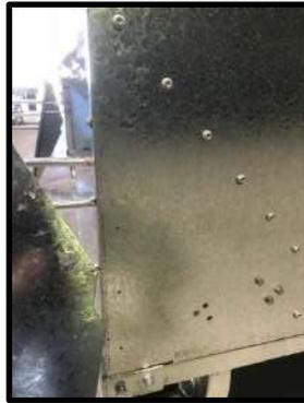
**STEP 5:** Don't tek screw this side of ends. This will be done when rain guards are fitted later.
