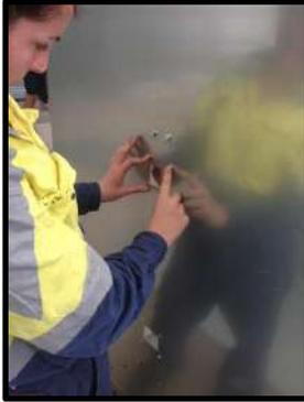
**STEP 16:** Fit sight glasses with small screws and nuts provided.
