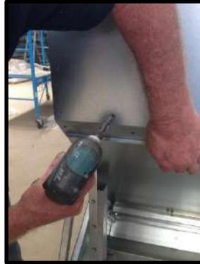
**STEP 65:** Second tek screw to be the second hole from the end (Do not do the hole at the end first).
